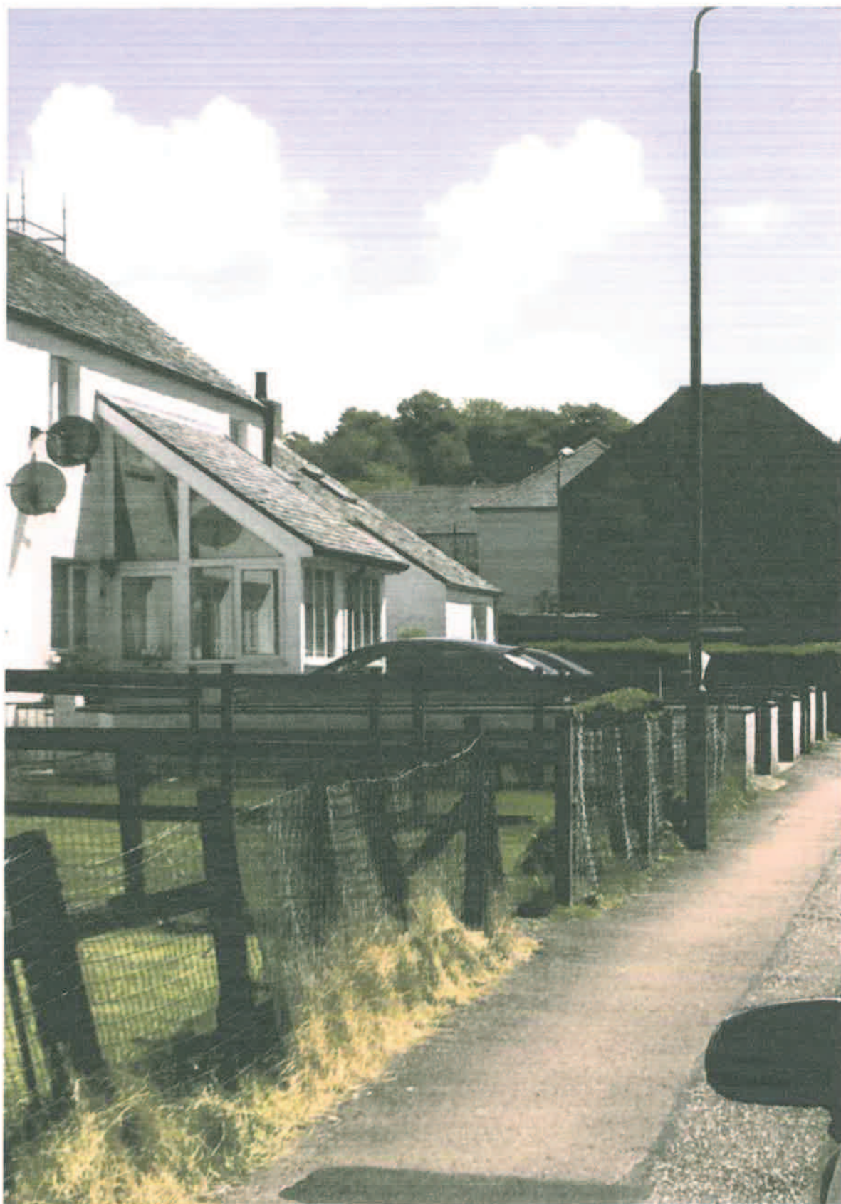
Porch Extensions in Union Street Lochgilphead which are larger than the proposed extension and which clearly overshadow the living room windows.
